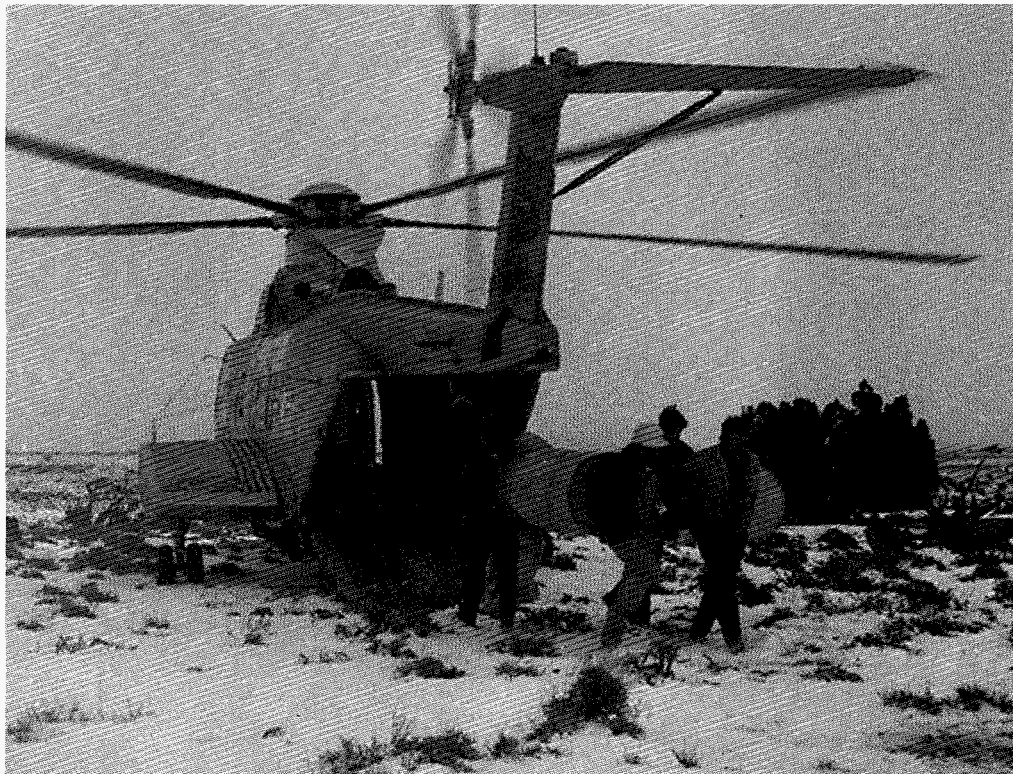
Test range maintenance crew delivers orange barrels by helicopter in May 1965 to mark the flight path for Joint Task Force 2 tests.
