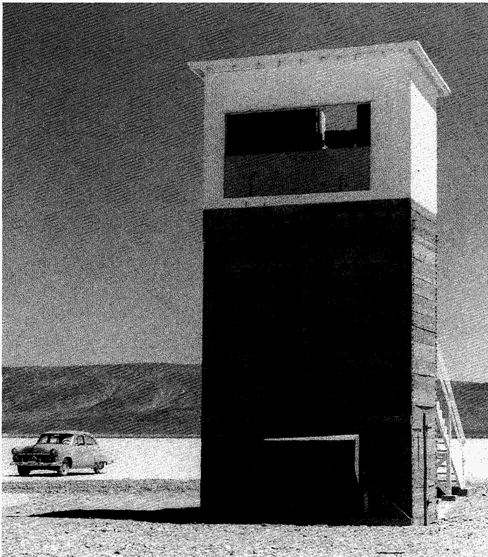
Cameras at Yucca Flat were elevated in this structure for maximum test coverage.
